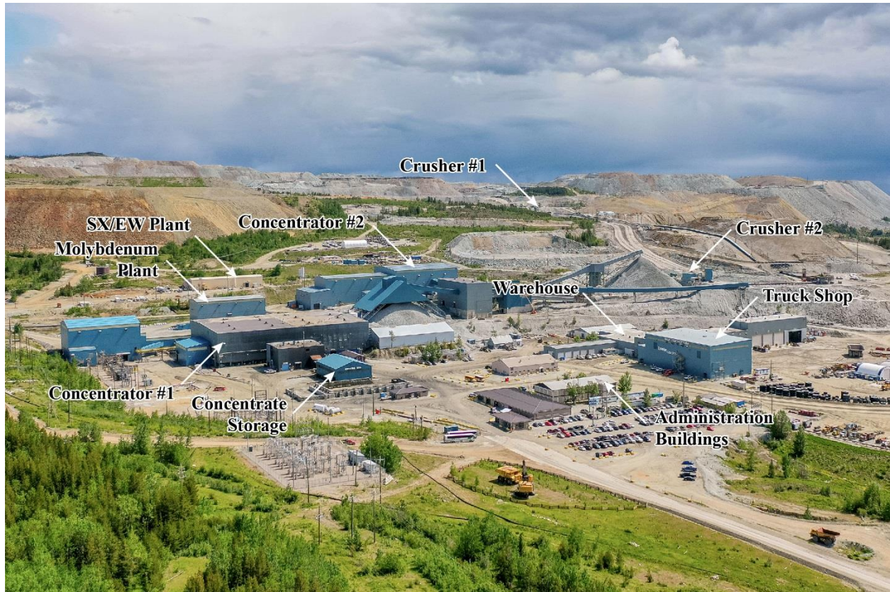
Figure 1-2: Plant Site Configuration
